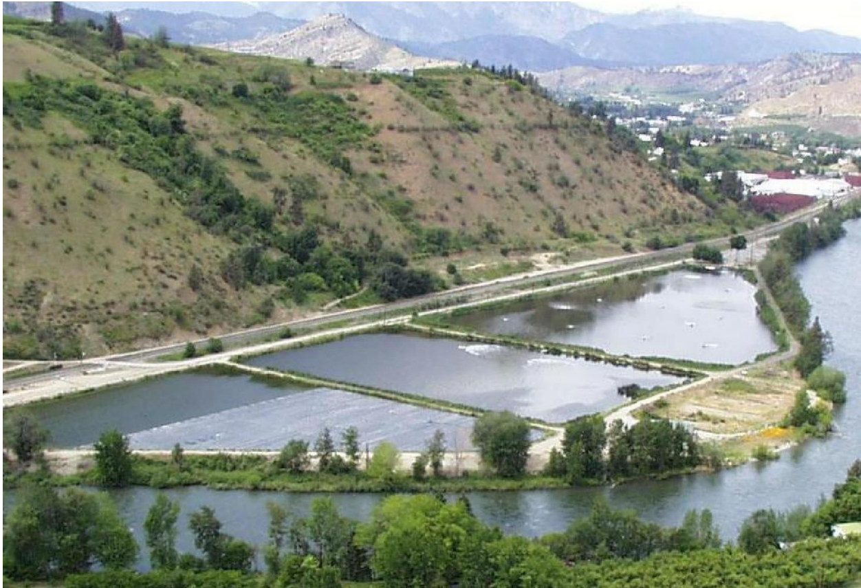
Exhibit 2.1. Former Wastewater Treatment Lagoons.
