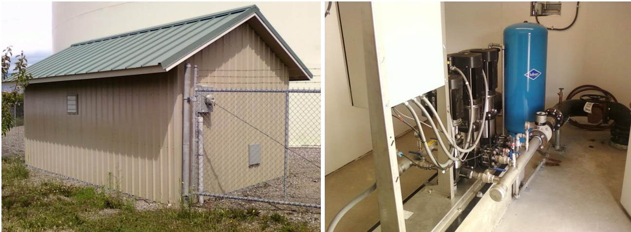
Photo 1-10 Vista Heights Booster Pump Station
