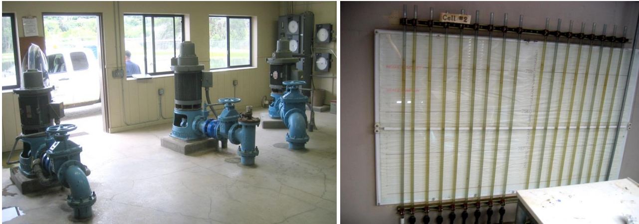
Photo 1-5 Water Treatment Plant Pumps and Cell Level Board
