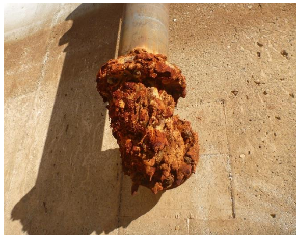
Photo 2: Existing Overflow Piping
