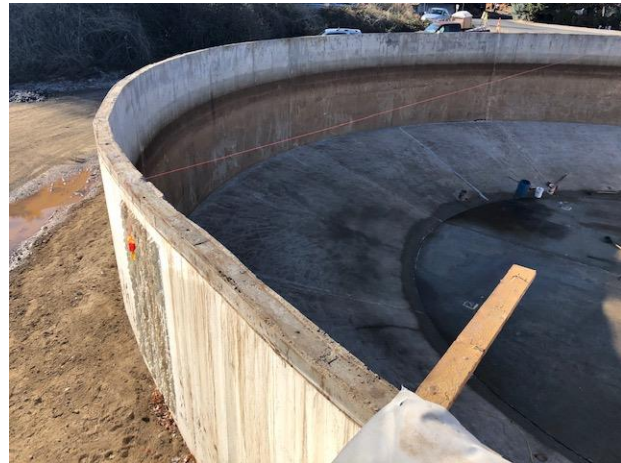
Photo 8: Existing Wall Exterior
