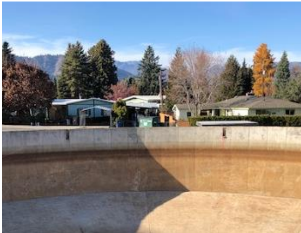
Photo 7: Existing Beam Seats
