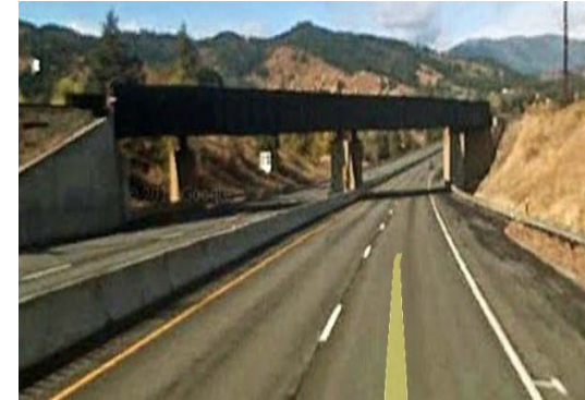
Figure 6.2: US 2 Railroad Overpass
